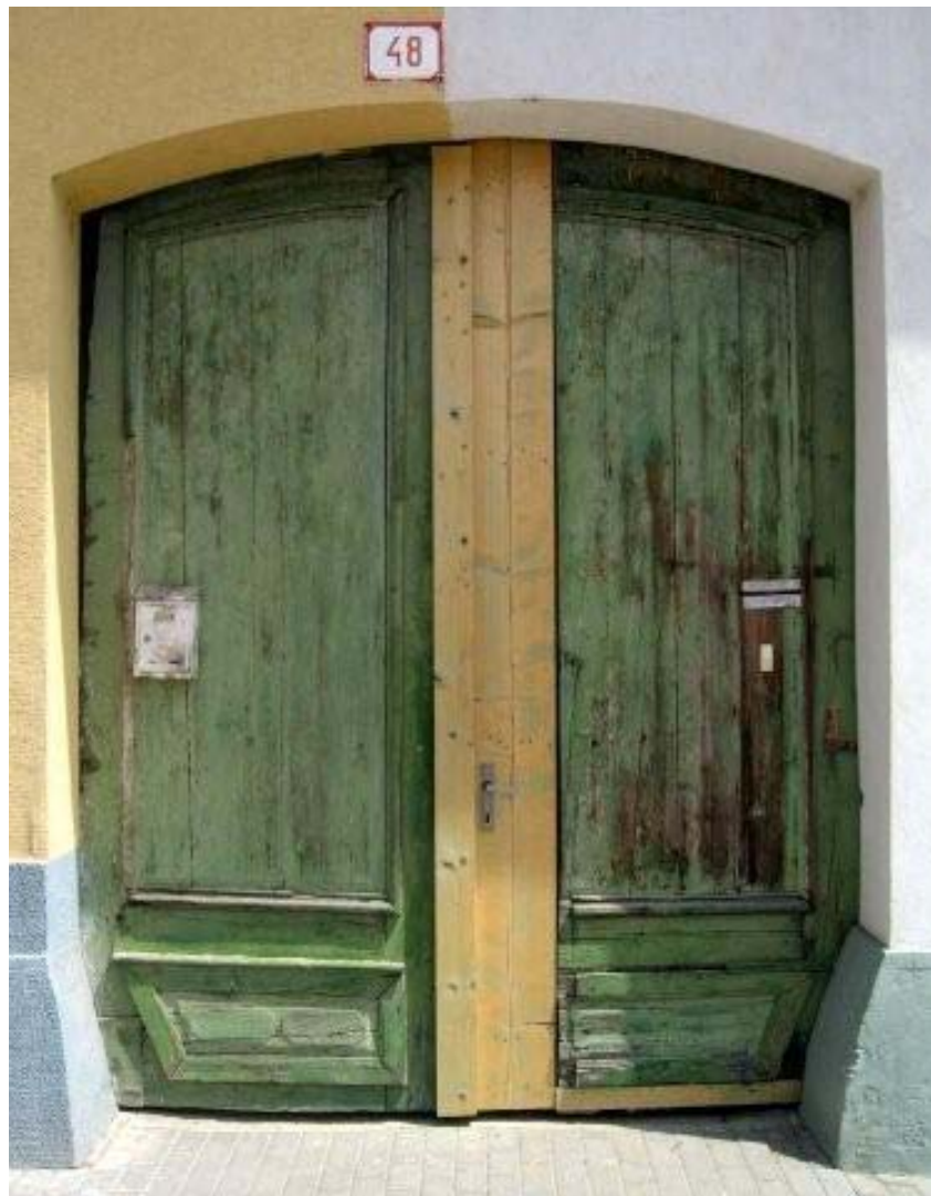
pic.29 the door in a process of repair rate
