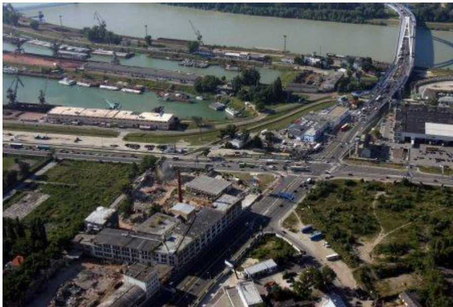
The arial view of lisovňa and the Košická street site before the demolition.
