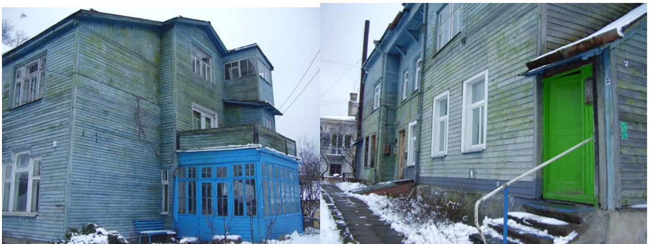
13 fig. Collective ownership “creates” a jazzy and patchy house face. Vytauto 34/Treniotos 1. Listed house. Reg. Nr. S-589. Built in 1901. Pušų 43/15. Listed, reg. Nr. S-622. Built in 1910.
