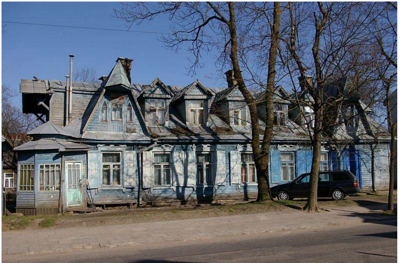
5 fig. Vytauto 49. Listed building, reg Nr. S-591. This house possesses a characteristic to Russian style form of gables. A slanting composition of consoles as well as a multangular veranda is projected according Swiss style.
