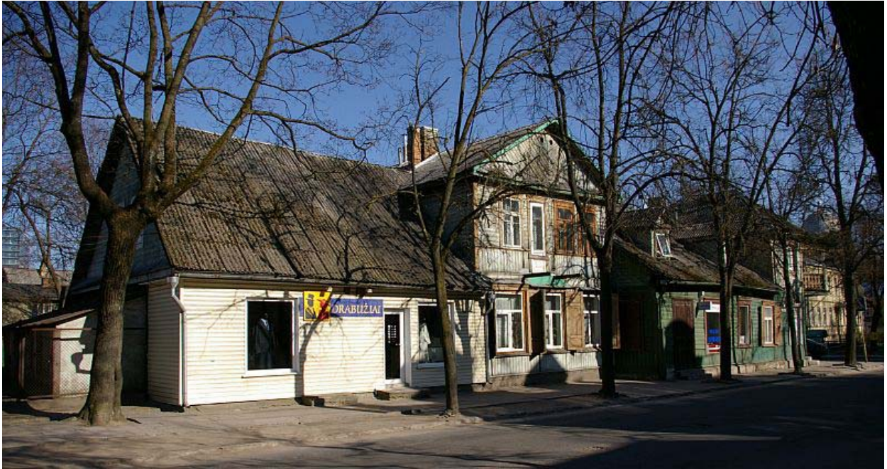
12 fig. A partly „restored“ house – a „beauty“ of plastic windows and plastic planks. Vytauto 37/Pušų 9. Listed house.
