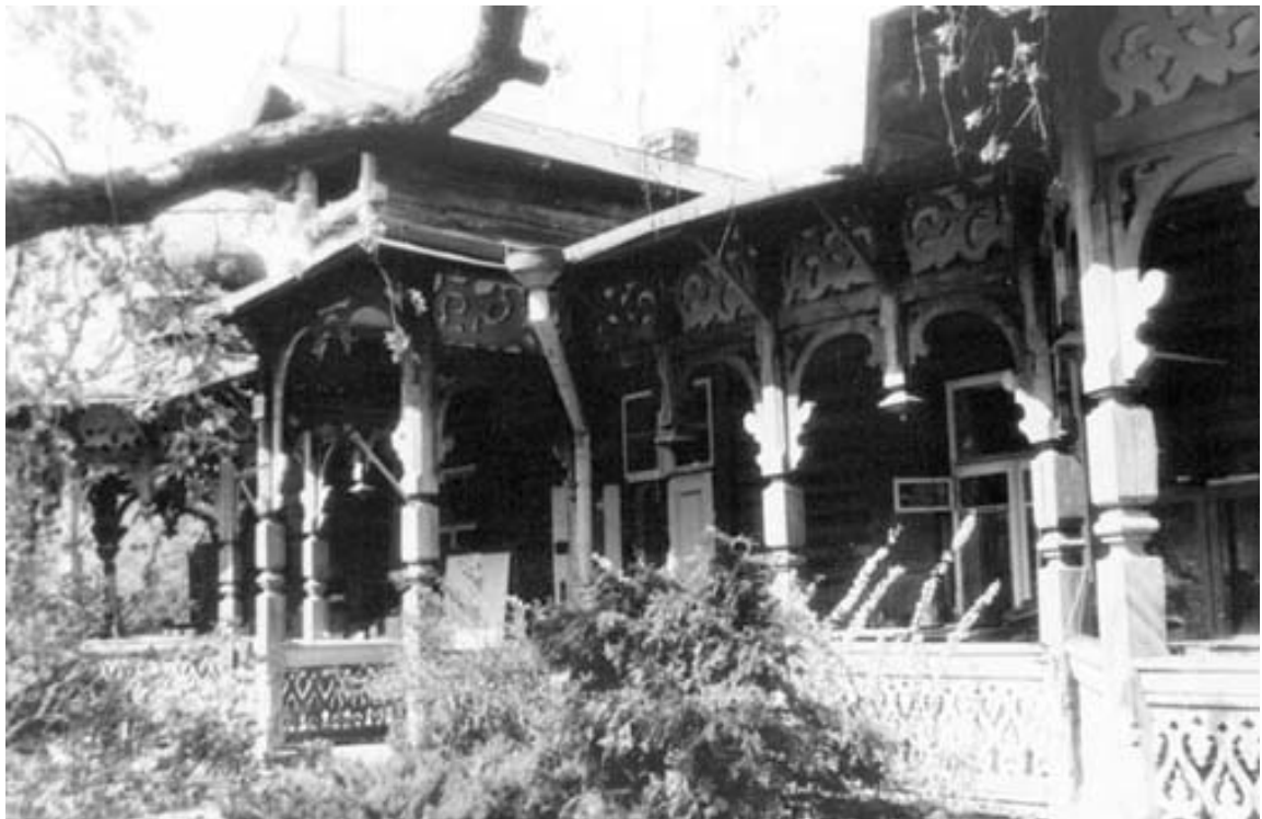
7 fig. More rare and unusual manifestations of historicism style remained in the suburb of Žvėrynas. This living house possesses the oriental, so called Mauritanian, motives: small arcs of horseshoe in the strips of décor, azure crosscut ornamentation of the fencing of veranda. Poškos 61. Listed, reg. Nr.S-574. Built in 1901.
